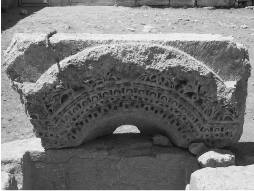
Fig. 2.5.7 Loose niche head close to the cathedral
